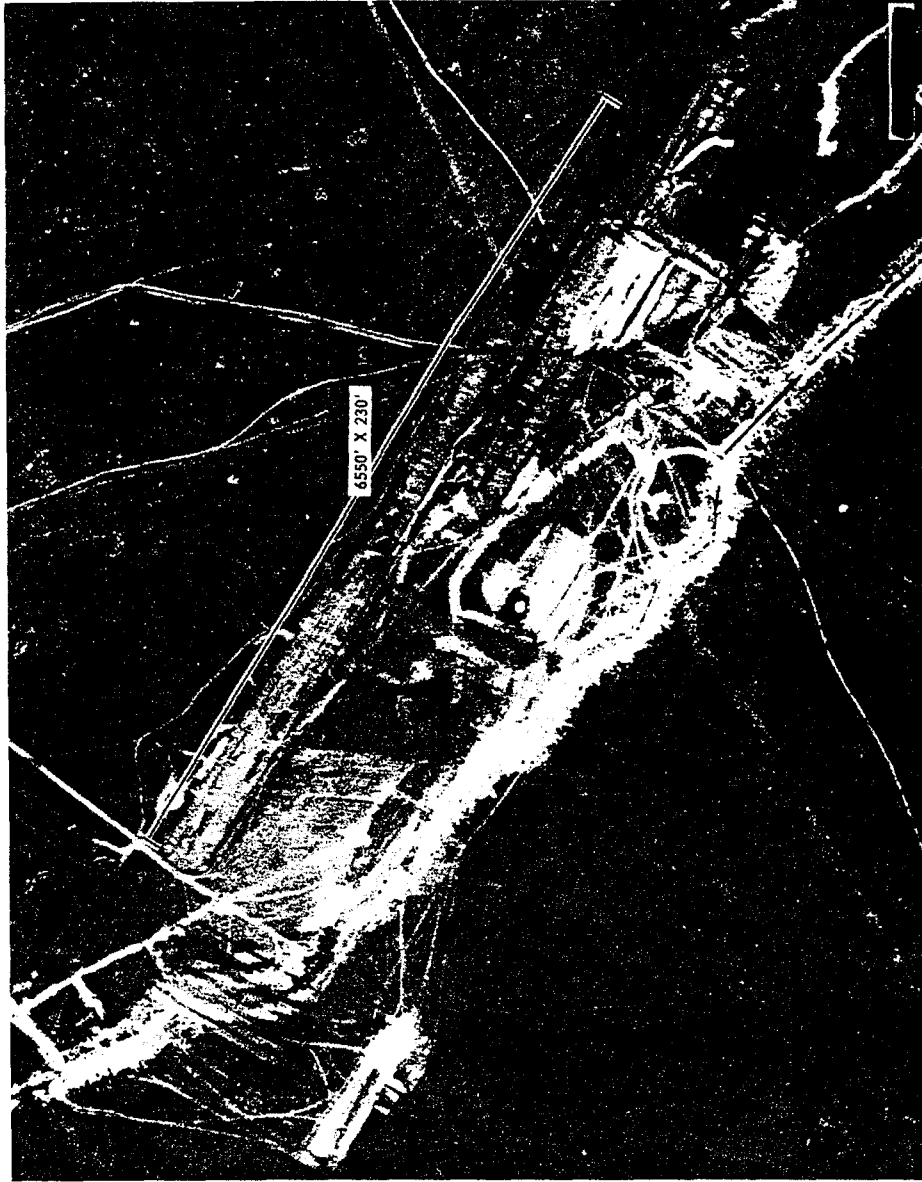
AIRFIELD UNDER CONSTRUCTION, CHOYBALSAN, MONGOLIA (AIRFIELD BONUS)
