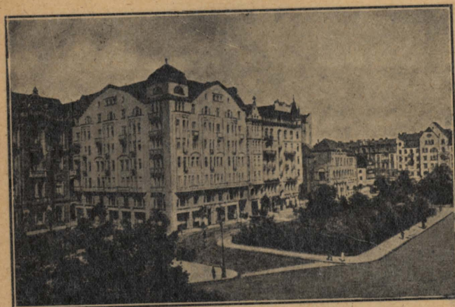
62. Napoleon's Square in Warsaw.
