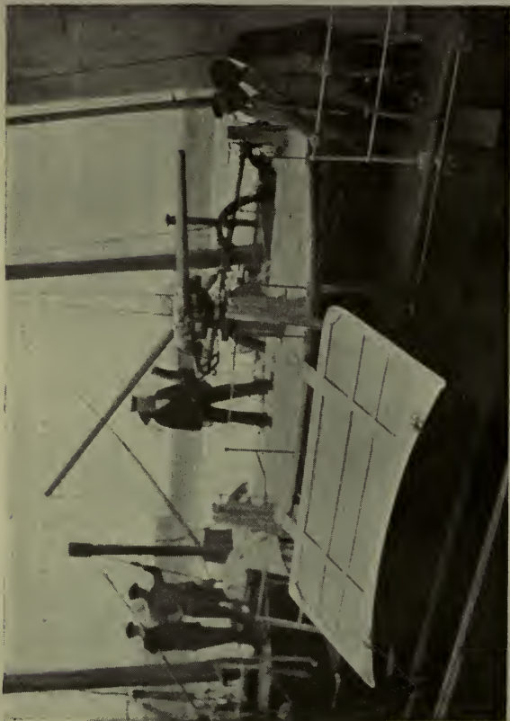
Sketch No. 2 (taken at 25 feet) shows the dummy davits down, the boat gone and the gun deck cleared for action within three seconds from the word of command having been given.
